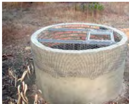
FIGURE 3. WELL COVERED WITH A METALLIC NET PROTECTED FROM THE ENTRANCE OF IBERIAN LYNXES. DROWNING IN WELLS WAS DETECTED AS A RELEVANT CAUSE OF MORTALITY DURING THE 90'S.
